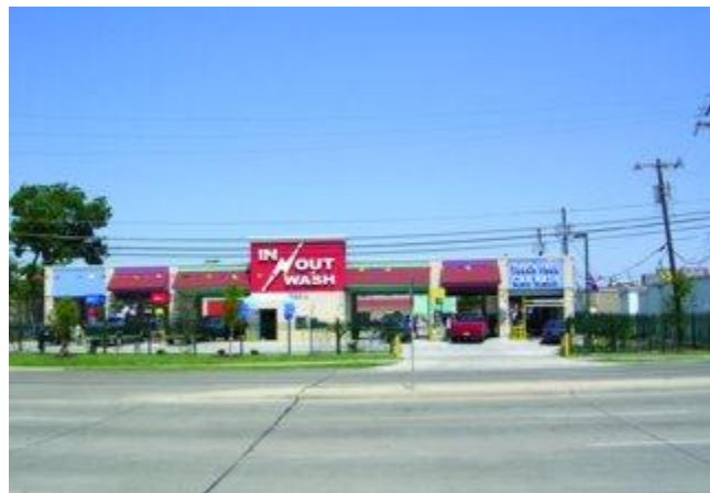
Street exposure serves as an invitation. Note the wrought-iron fence.
